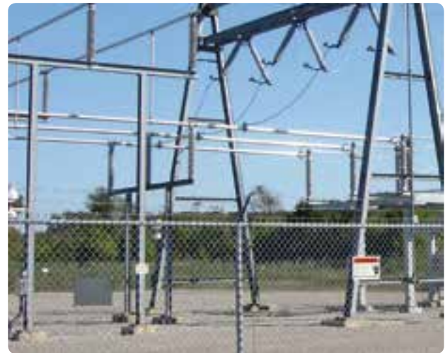
Figure 15 A 132 kV disconnect switch
