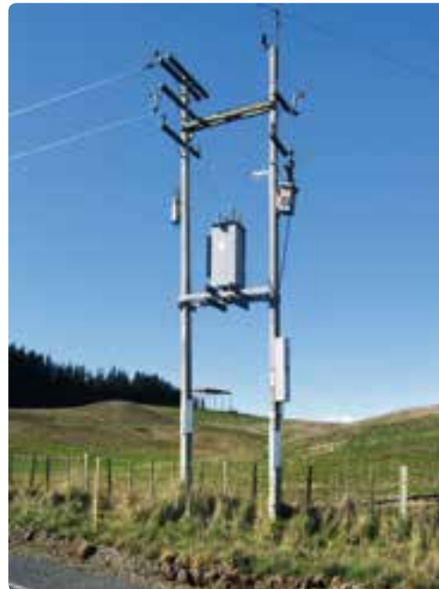
Figure 6 SWER isolation transformer and take off line in New Zealand
