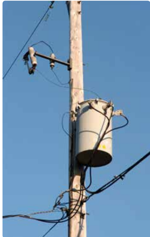
Figure 1 Single Phase Transformer used in Bangladesh
